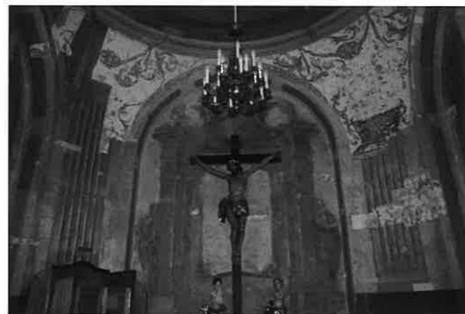
Fig. 7. Smogorzów, a fragment of the illusionist altar in the Holy Cross chapel with extensive exposures of the former decorative layer Source: author, 2017
